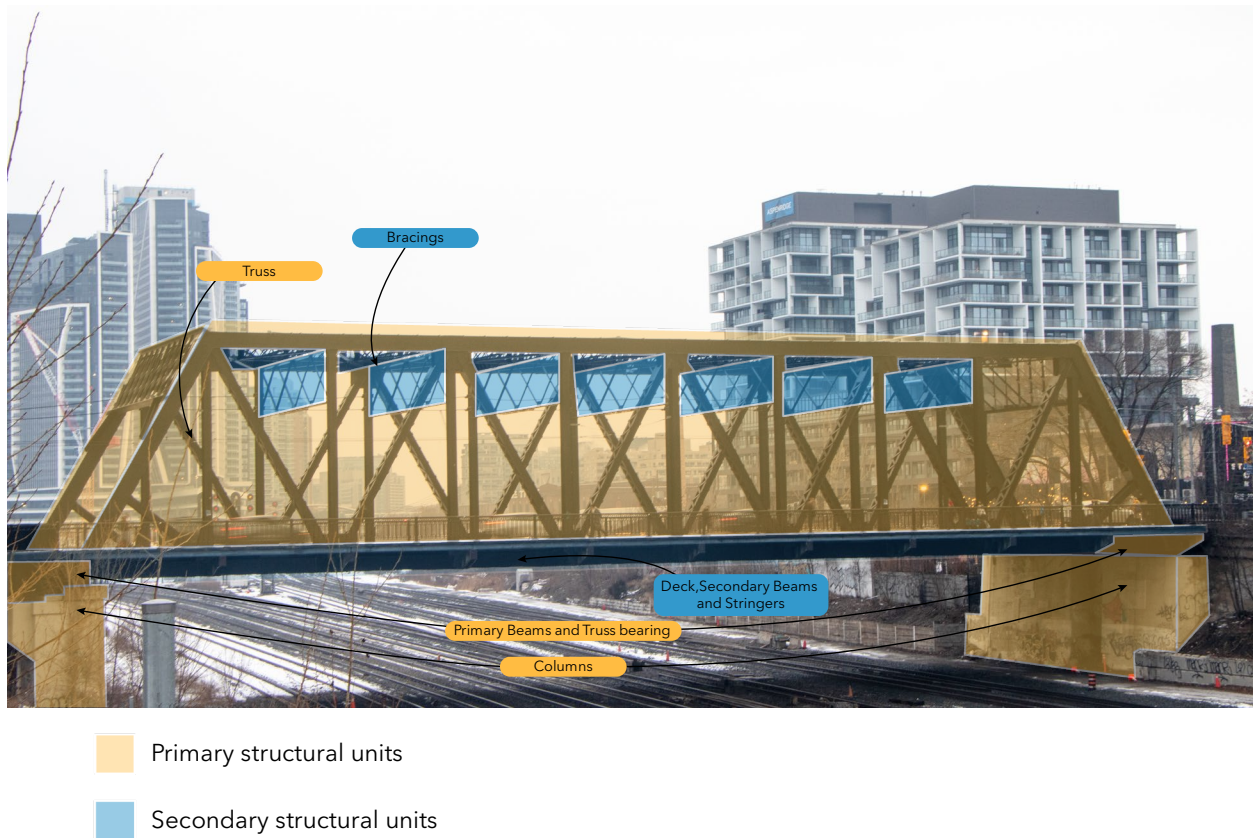
Figure 2 Illustration of structural hierarchy | Image: Léo Trédille 2025. CC BY-NC
