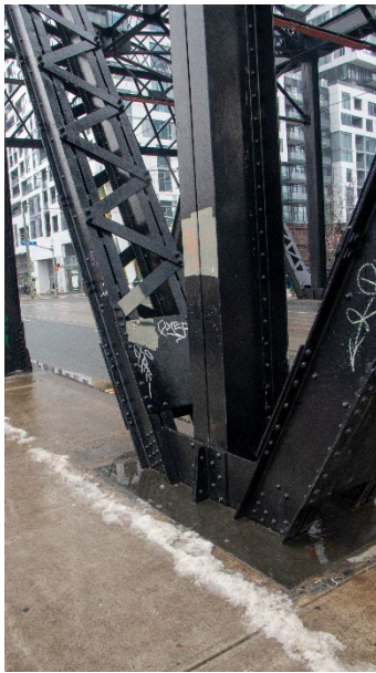
Figure 5 Joint between truss and beams | Image: Léo Trédille 2025. CC BY-NC
