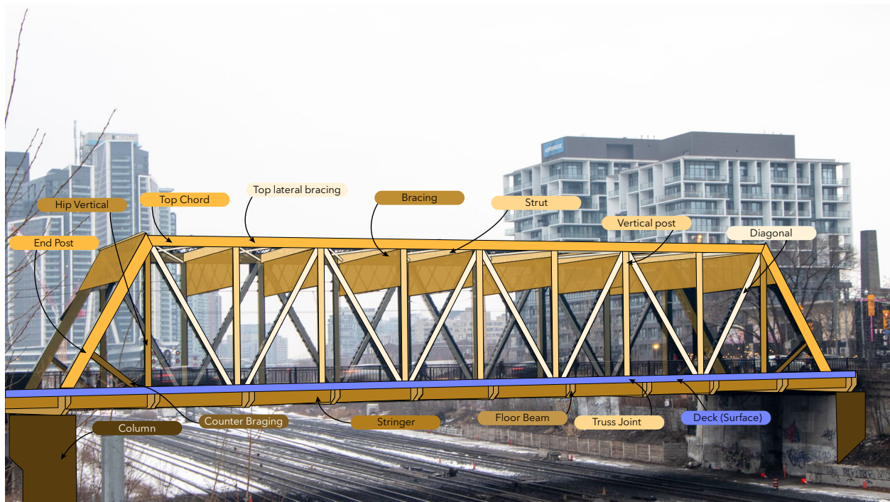
Figure 3 Illustration of structural elements | Image: Léo Trédille 2025. CC BY-NC
